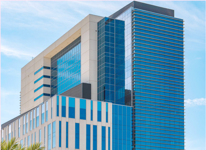
The different heights, modulation and materials create a distinctive massing for this building.
