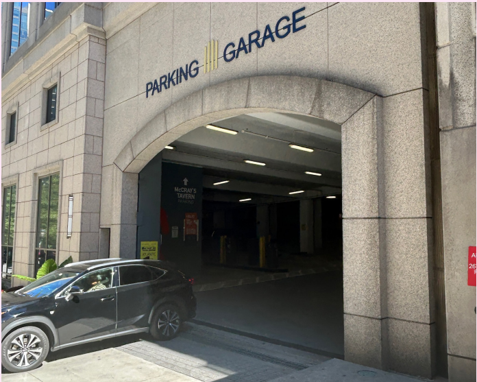
This building has appropriate integration of vehicular entry with building architecture.
