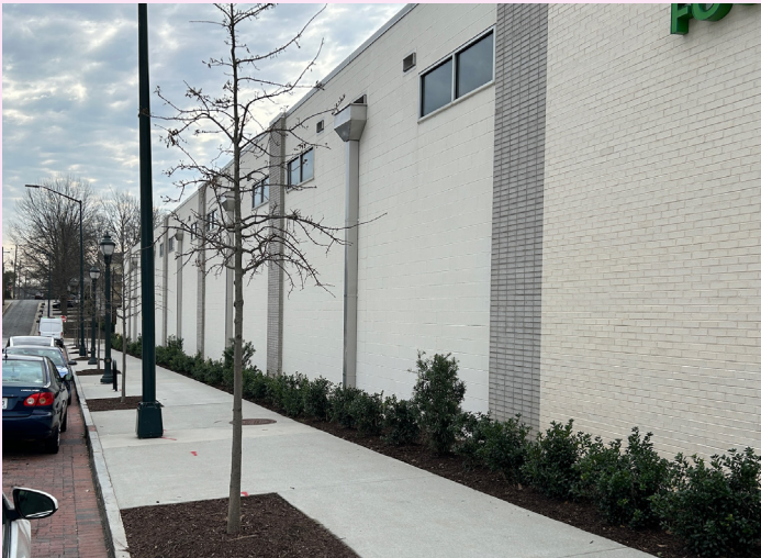
Ground floors should activate the streetscape, in no case should blank walls such as this be proposed in downtown.
