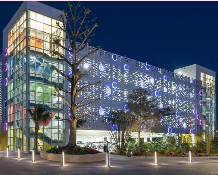
This parking garage has landscaping on the ground level and a playful perforated aluminum pattern on the upper levels helping screen the vehicles from the public realm.
