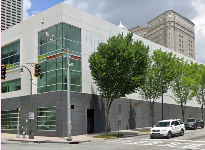
This building lacks façade continuity, creating an uninviting street frontage.
