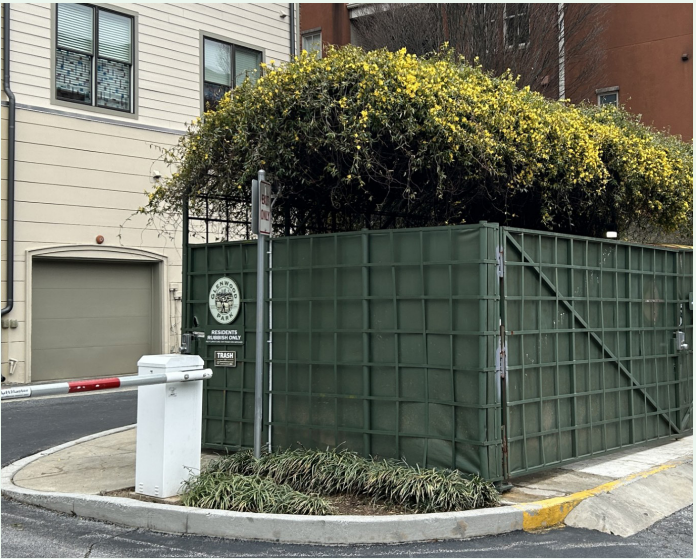
This enclosure incorporates a trellis so equipment is less visible from upper floors.
