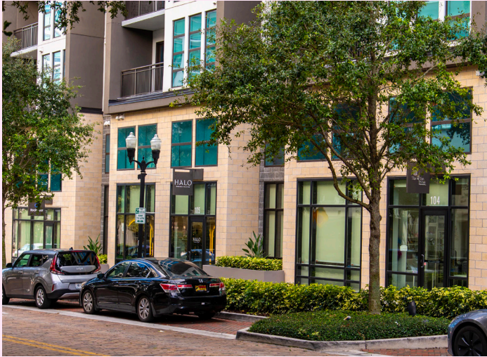
The fenestration patterns and depth break down the horizontal scale of the building base.
