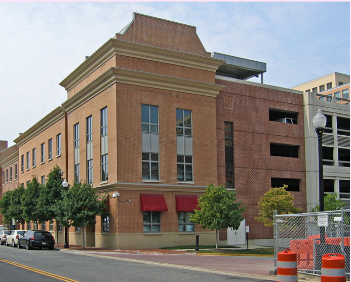
Three floors of active use is provided to screen this parking structure.
