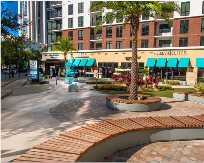
This building incorporates a plaza with outdoor space and sitting areas.
