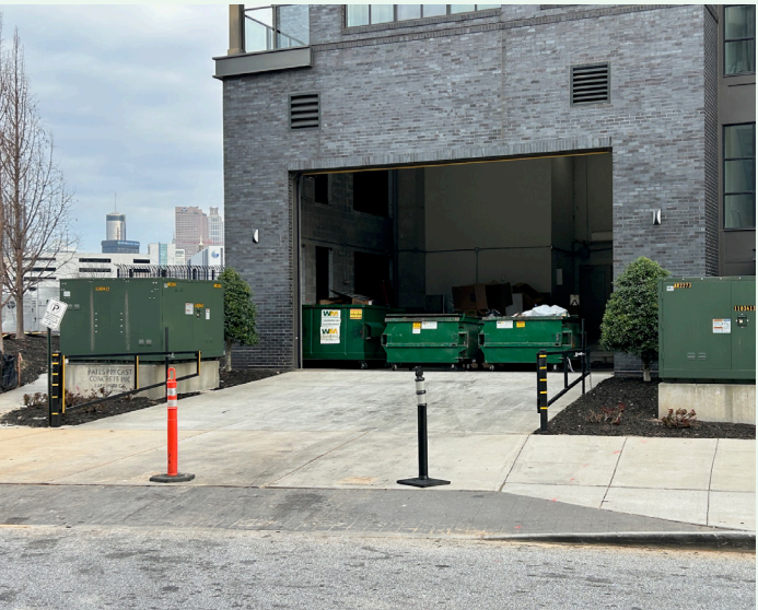
The placement of the service bay creates an unnecessarily wide curb cut that impedes the pedestrian zone.
