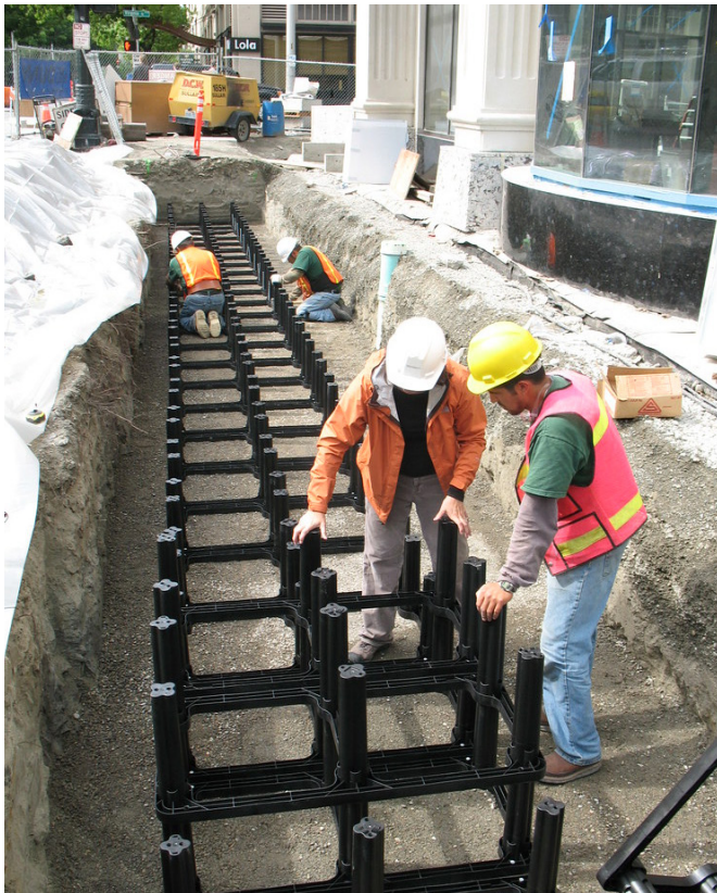
Soil Cell Installation (Source: https://www.deeproot.com/products/silva-cell/ )
