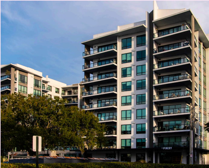
Articulation is well scaled for each portion of the structure providing façade continuity and depth.
