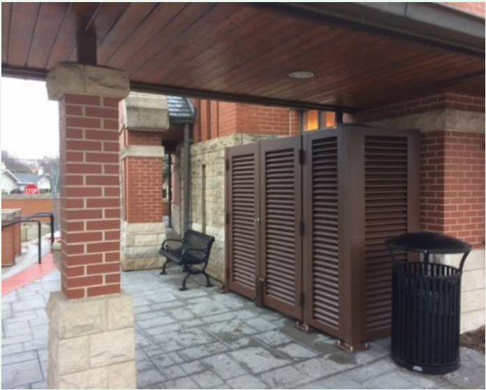
Screening is incorporated as an extension of the building, using a color and material palette that effectively blends into the environment. (image credit: PalmSHIELD)
