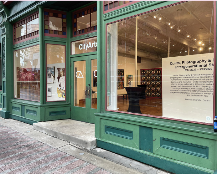
Large windows provide views into the storefront, and a setback entry with glass doors is also provided to avoid interrupting the sidewalk.
