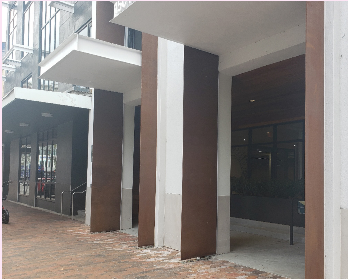
The colonnade shown above is not designed as an extension of the sidewalk zone and encourages hidden activities.
