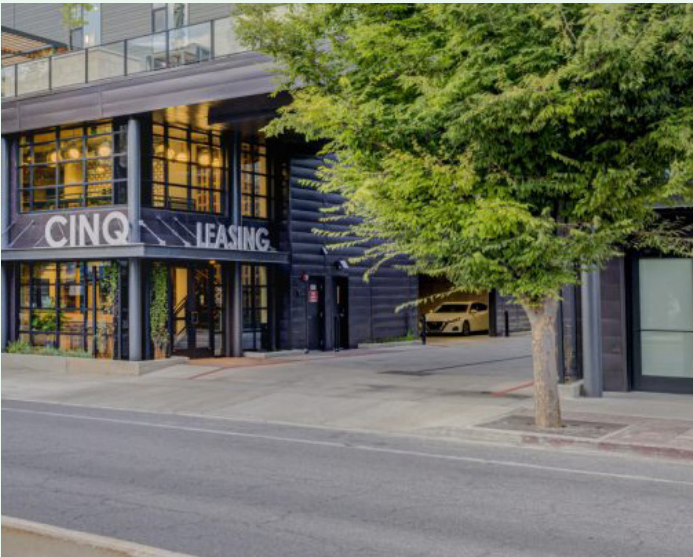
This curb cut provides access for both parking and service internal to the site without creating a break in the sidewalk.
