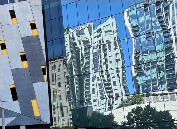
The reflective glass used on this façade creates a singular mass without any depth.
