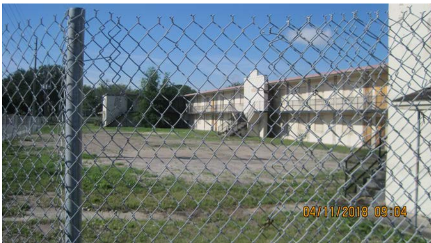
Photo #9 - Looking at apartment building at 800 South Tampa Avenue from the intersection of South Tampa Avenue and Orange Center Boulevard
