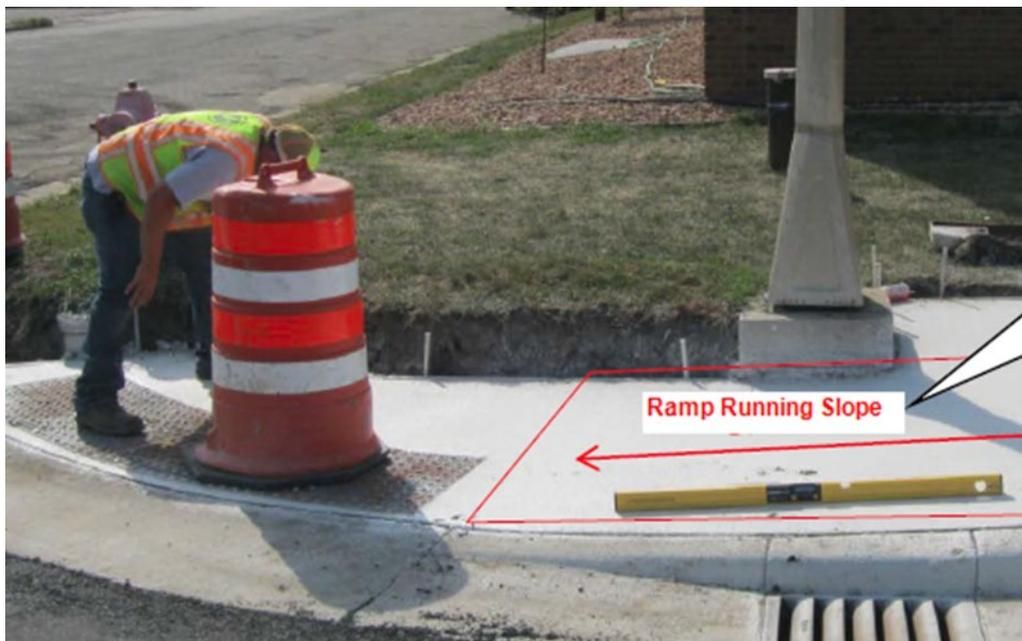
The PROWAG Guidelines Sections R304.2 – R304.4 specify a maximum allowable running slope of 8.3% and a minimum allowable running slope of 5% for compliant curb ramps. Section R304.5 of the same Guidelines specifies a maximum allowable cross slope of 2%.
