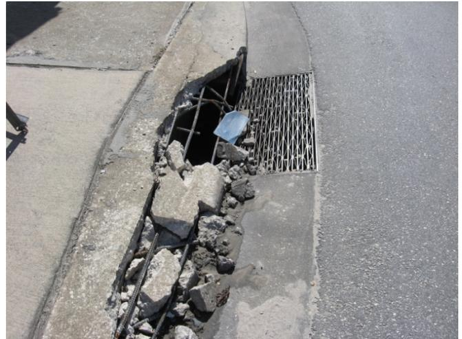
*Fig. 15.* Damaged curbs need maintenance.
