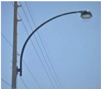
The Sole City Luminaire can be bracket-mounted to existing utility poles as shown with this alternate (comparable) fixture on Orange Blossom Trail
